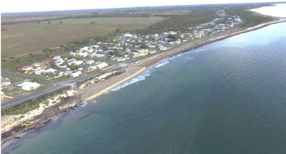
Figure 2: Southern (top) and northern (bottom) reach nourishment photographs (KDC 11 June 2020)
