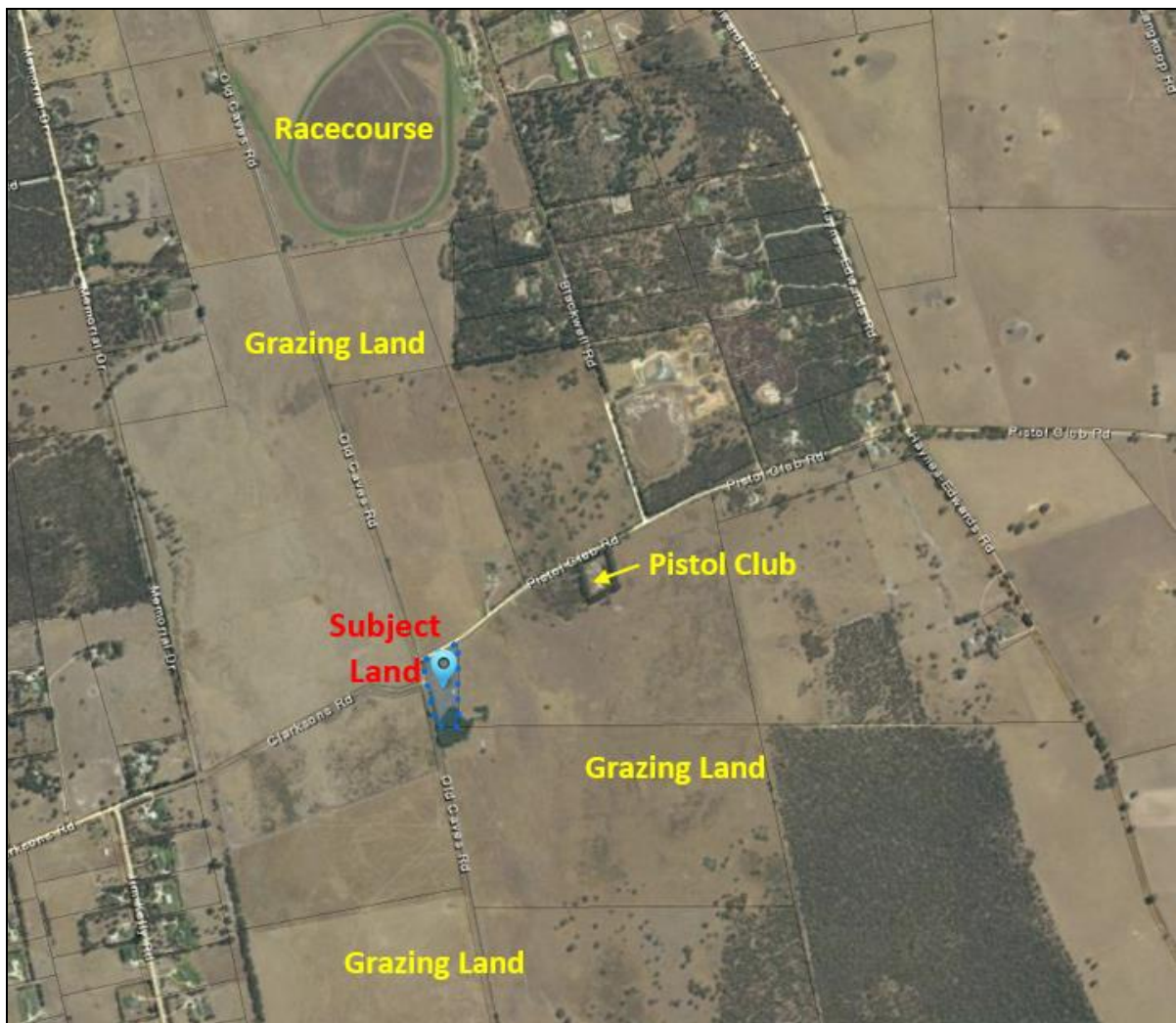
Photo 7 – aerial photograph showing the landuses existing in the general locality around the subject land.
