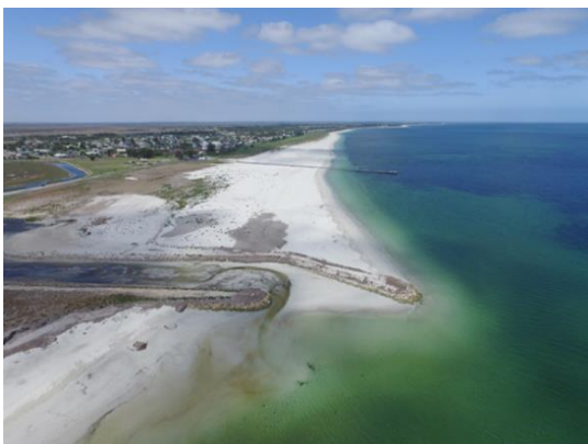
Photo: Maria Creek breakwater January 2020
