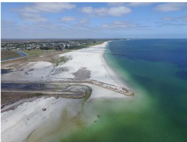
Photo: Maria Creek breakwater January 2020; sand accumulation to full length
