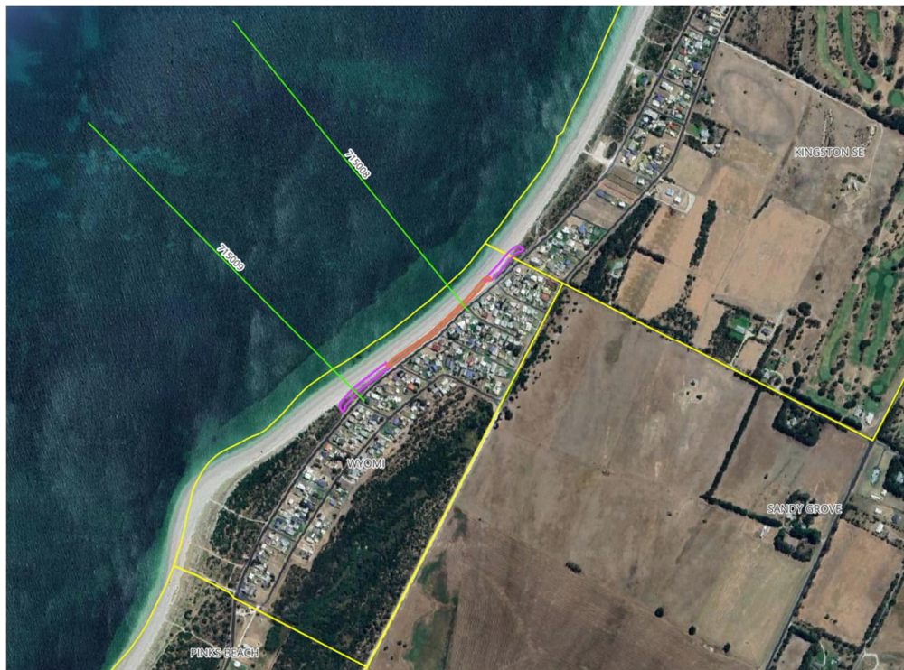
Figure 2-2: Existing DEW Profiles (Green Lines), Seawall Stage 1 (Orange Lines) and Stage 2 as-Constructed Seawall Extension (Pink Lines) at Wyomi Beach
