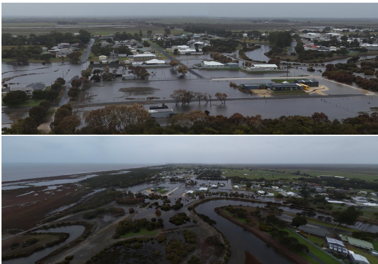
Figure 1.1 Photos from recent storm surge event in Rosetown
